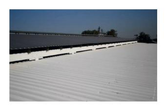
When applying the product with a brush, it is necessary to apply three cross layers to ensure adequate protection.
